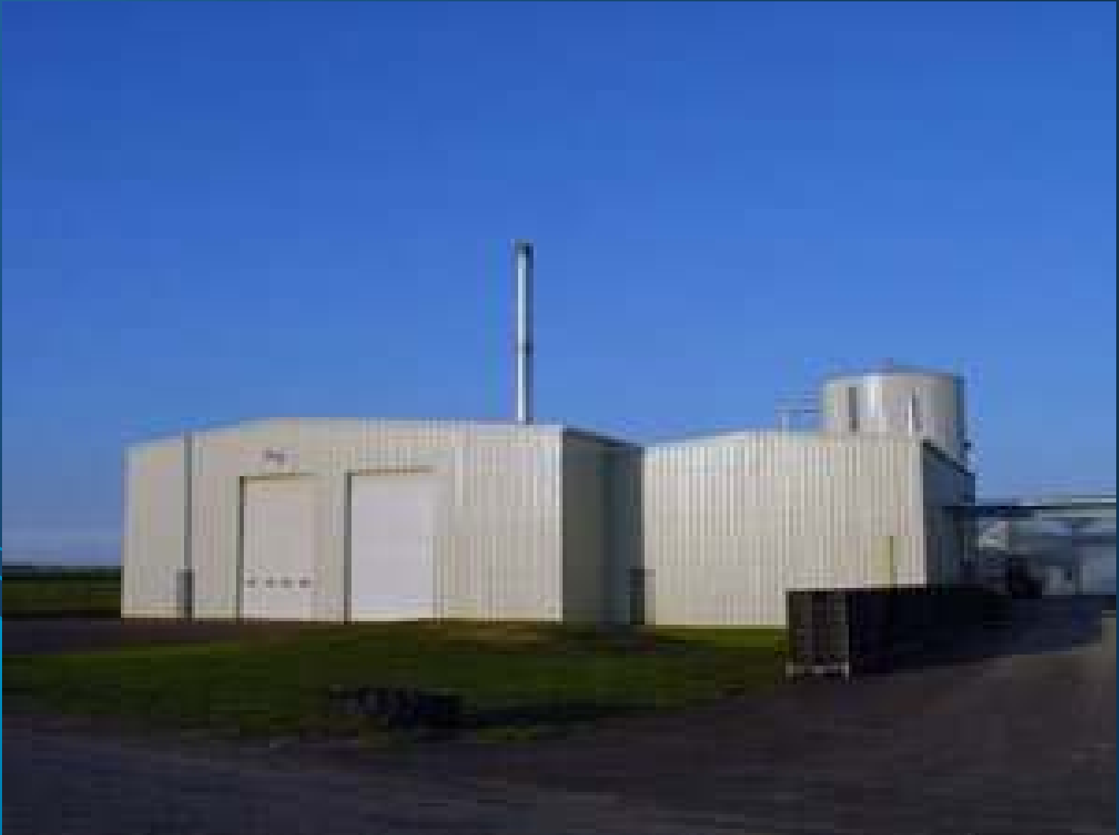
Wood chips and barks gasification plant, Foothill Greenhouses, Ontario (CANADA)
